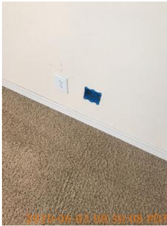
2020-06-03 08:30:08 PDT Switch/Outlet 📅 2020-06-03 08:30:08 🔍 32.91316596450838, -96.86307711887466 🖼️ Image
